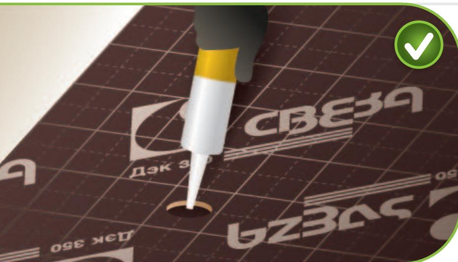
Fill all holes, made in the course of installation works, with a silicone-based adhesive to prevent penetration of moisture (swelling).
