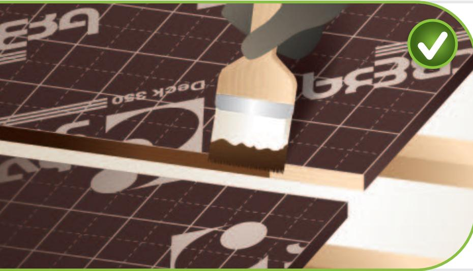
When cutting plywood, protect flat ends with paint. SVEZA recommends to use the acrylic paint **TEKNOS Teknol JRL** (Finland) or a sealant to prevent penetration of moisture (swelling).
