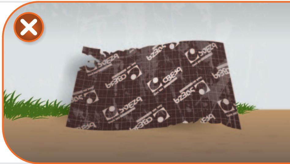
Plywood sheets, intended for assembling of the formwork on the following floors, should be arranged to be hoisted by a crane to the floor above.
