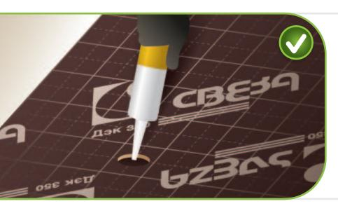
Fill all holes, made in the course of installation works, with a silicone-based adhesive to prevent penetration of moisture (swelling).
