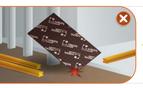
Avoid dropping plywood and dragging it over the ground.
