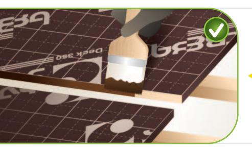
When cutting plywood, protect flat ends with paint. SVEZA recommends to use the acrylic paint TEKNOS Teknol JRL
